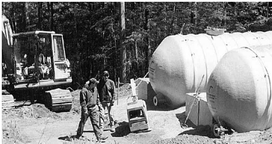
Shawn Tryon and Keith Amstead during the installation of the two 10,000 gallon storage tanks above the Monterey Water Company's pumphouse off Sandisfield Road.
