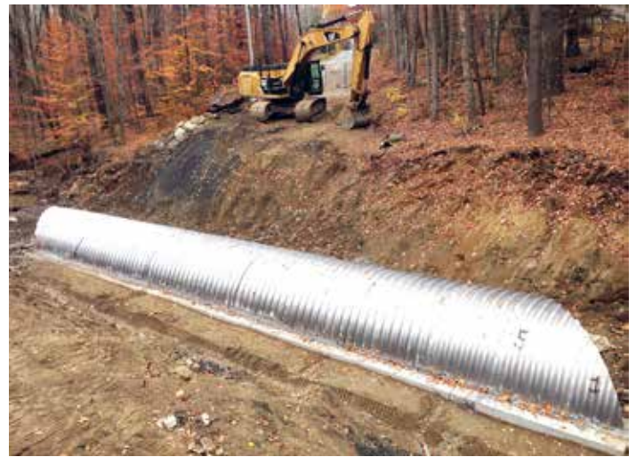
Two large excavators working on rebuilding the Tyringham Road culvert. Director of operations Shawn Tryon was working the larger excavator with Tryon Construction assisting. The new heavy-gauge aluminum culvert is nine-and-a-half feet wide at the base, and seventy-three feet long. —Photos by Stephen Moore
