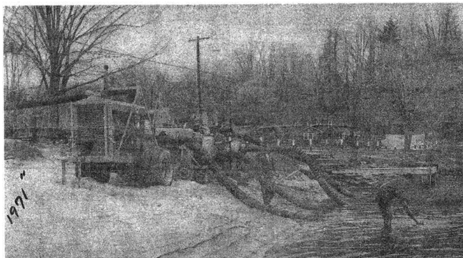
DIESEL-POWERED suction pumps suck water from Lake Garfield and push it through pipes at left to downstream side of dam whose reliability has been questioned by county and local officials. The pumps are manned 24 hours per day by workers from the Perini Corp. of Framingham under contract with the Army Corps of Engineers. Deane Hulick
