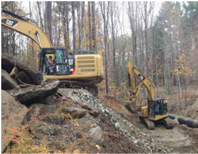
Two large excavators working on rebuilding the Tyringham Road culvert. Director of operations Shawn Tryon was working the larger excavator with Tryon Construction assisting. The new heavy-gauge aluminum culvert is nine-and-a-half feet wide at the base, and seventy-three feet long. —Photos by Stephen Moore
