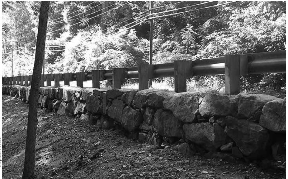
Sections of the large stone retaining walls being built by Palmer Paving on the steep downhill slopes alongside Route 23
