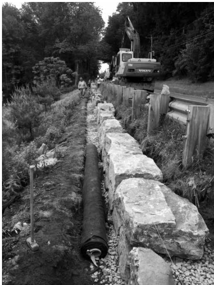
Sections of the large stone retaining walls being built by Palmer Paving on the steep downhill slopes alongside Route 23
