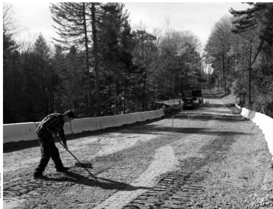
Shawn Tryon, director of operations, doing the final smoothing in preparation for paving.
