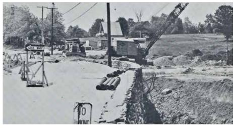
This construction photo shows the curved wall of the old dam and the old Tyringham Road. The roadbed for the rerouted Tyringham Road, and causeway over the equalizer pipes, is being built at the right.
