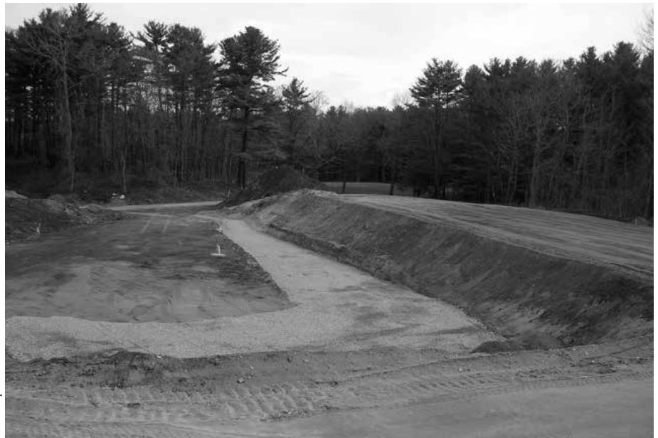
The new transfer station initial excavation and site work was completed by Tryon Construction during the third week in April. The open field pictured at center-right is a Gould Farm field on the far side of Gould Road. The elevated areas are for vehicles, and the lower areas for the compactors and dumpsters. The town anticipates the concrete forms to be assembled in place by mid-March.
