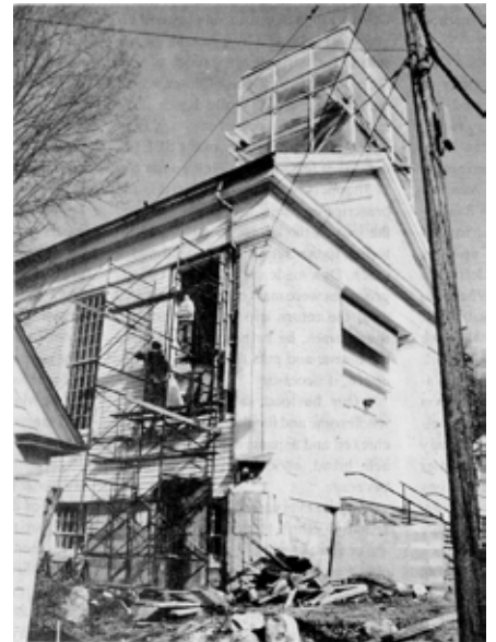
Kurt Hoelter and company prepare to install a new sash on the west side of the church. — Photo by Wayne Dunlop
