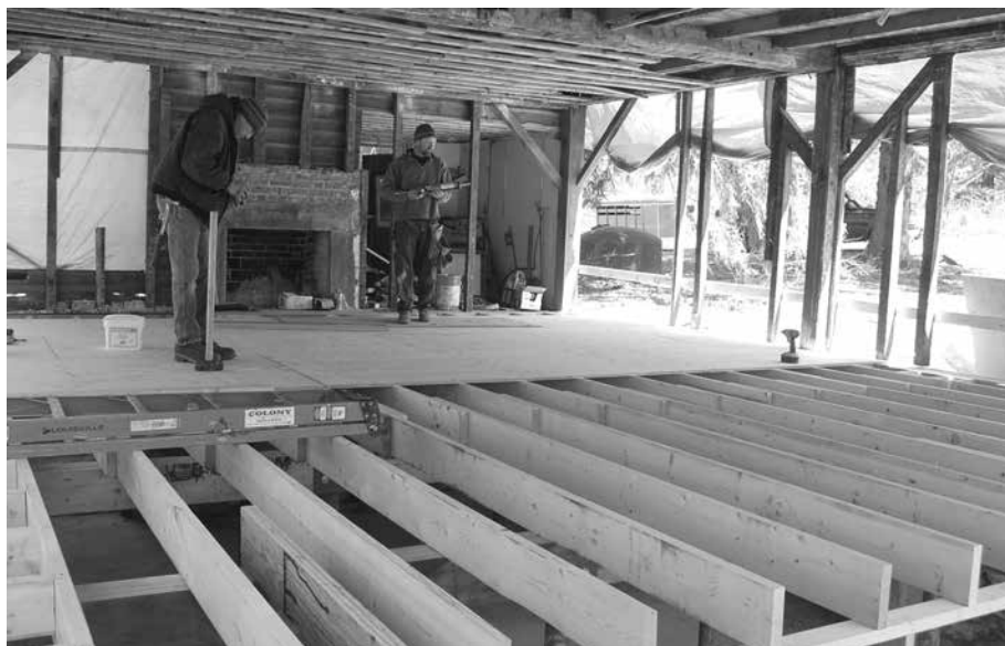
The new floor structure for the Wilson McLaughlin House is now complete. In this photo, Don and Troy of Kronengerger & Sons Restoration are installing the plywood subfloor. Stop by and walk around!
