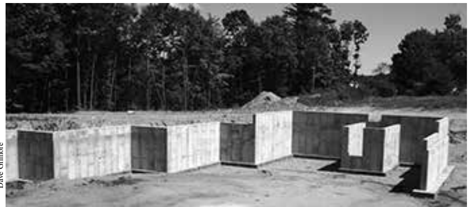
Transfer station concrete foundation is curing before being backfilled in early July.
